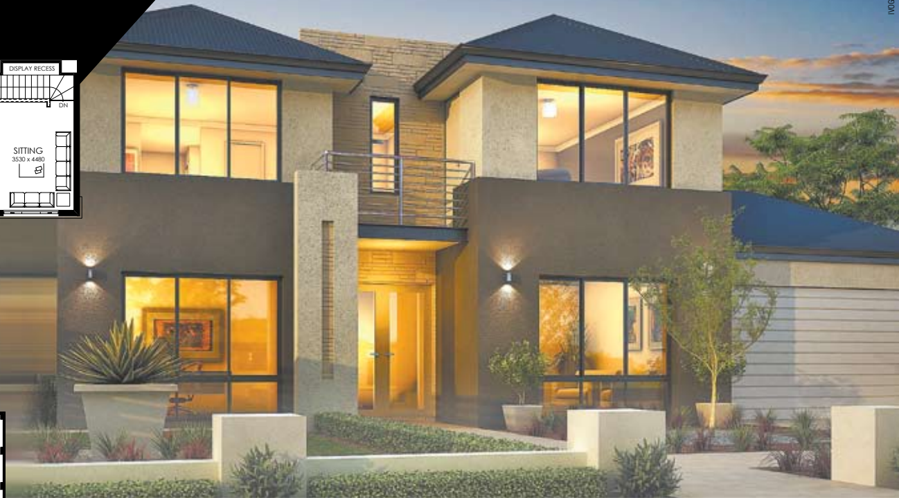
The Grant, $343,845. Includes elevation and floor plan as shown and specifications as listed below.
